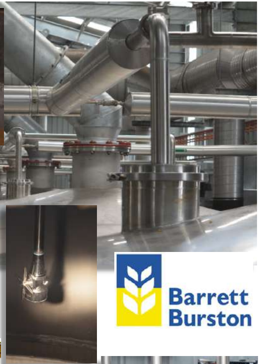
Designed and Installed of 12 x Toffejorg TZ 79 cleaning heads into Steeping Vessels.
