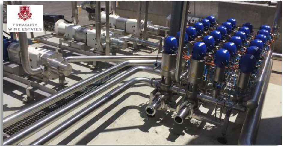
VALVE MANIFOLD DESIGN AND CONSTRUCT
